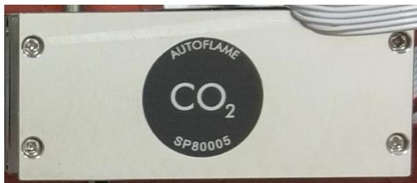
Figure 3.8.3.i CO<sub>2</sub> Cell
